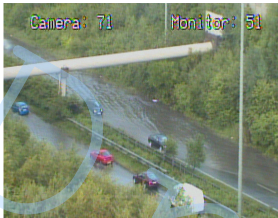
Figure 1 – Example of flooding on M50 orbital motorway around Dublin
